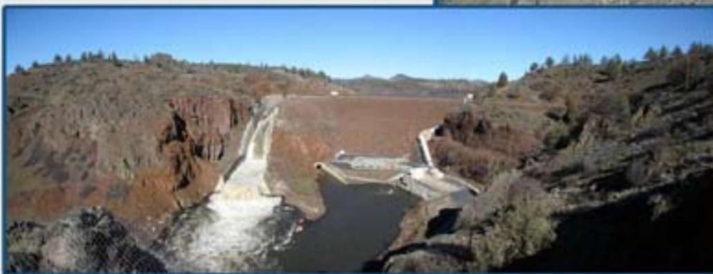
Iron Gate Damn
