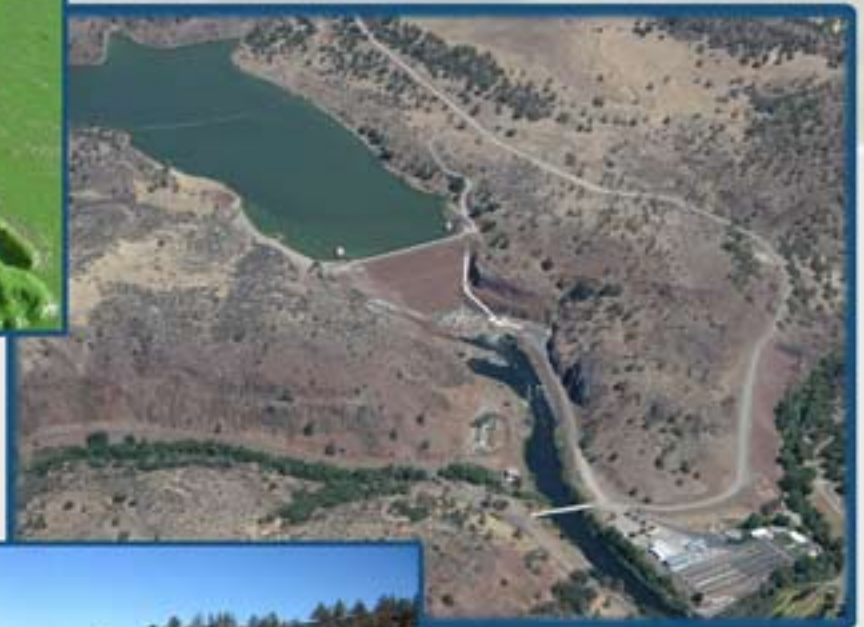
Aireal View of Iron Gate Dam
